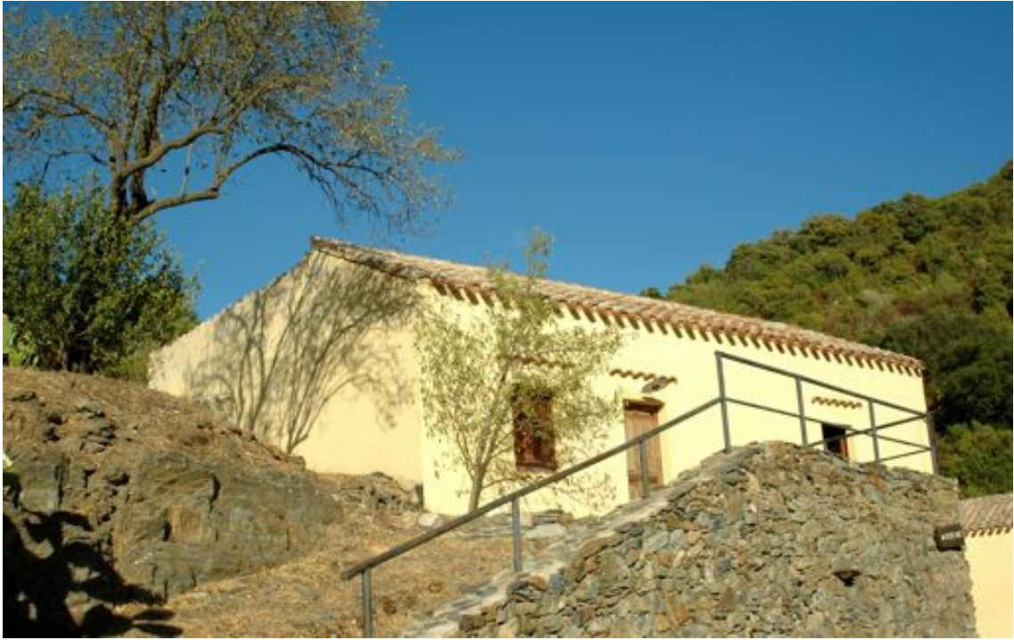
foto 7: a miner's house renovated and transformed into a residence
