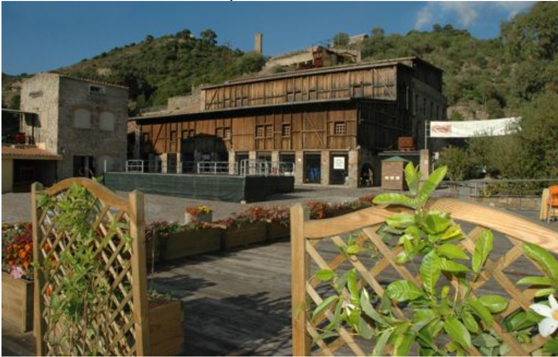
photo 1: Rosas washing plant
