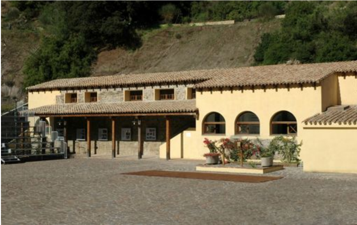
photo 2: the former chemical laboratory
